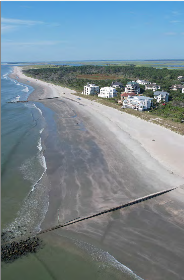
FIGURE 4.18. Groin #2 oblique aerial, July 2025. Much of the structure exposed above MLW.
