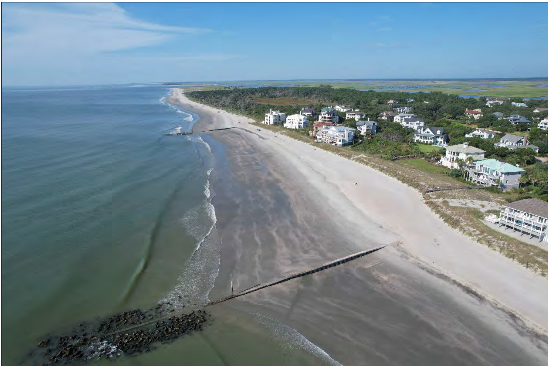
FIGURE 4.13. Reach 4 extends from the southernmost groin (background) to the central groin (foreground).
