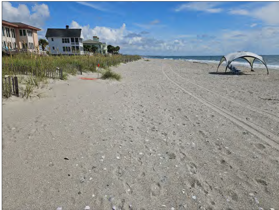
FIGURE 4.20. Between May 2022 and July 2025, the berm width in Reach 5 decreased by nearly 200 ft but these losses were partially balanced by volume increases along the submerged portion of the profile. Beach widths remain over 100 ft greater than the pre-project condition as of July 2025.
