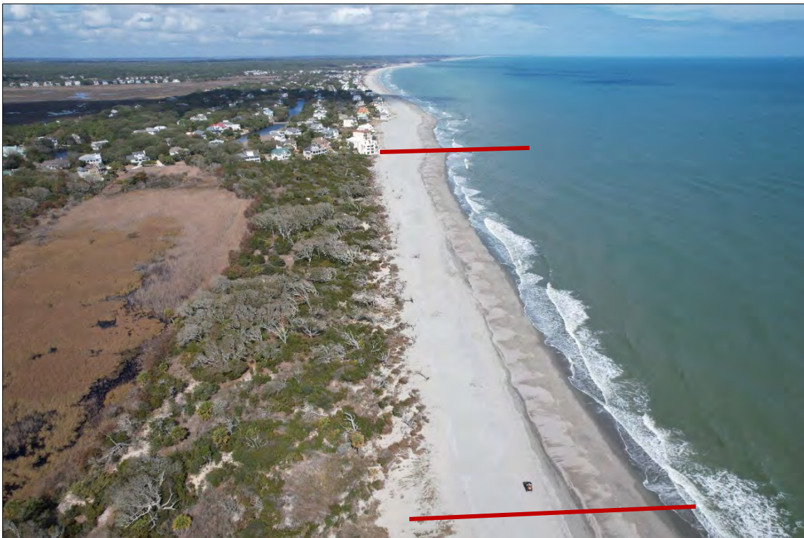
FIGURE 4.10. The North Hobcaw Reach extends from the central portion of the Hobcaw Tract (approximately 1,800 ft south of the southernmost groin) to the southernmost groin (highlight).
