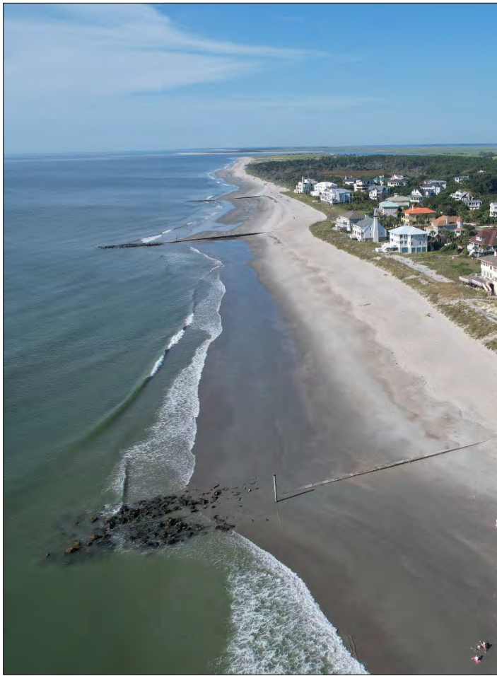
FIGURE 4.21. Groin #1 oblique aerial, July 2025. Much of the structure remains buried above MHW, allowing beach access alongshore at all tides.
